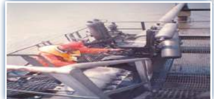
Actuator Change out at NGC/Ibom Power Plant Facility
