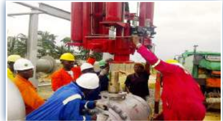
Actuator Change out at NGC/Ibom Power Plant Facility
