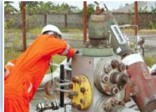
Christmas Tree Servicing/Maintenance
