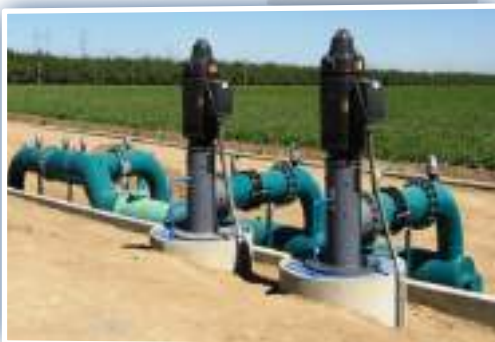
Pump Used for Crop Irrigation
