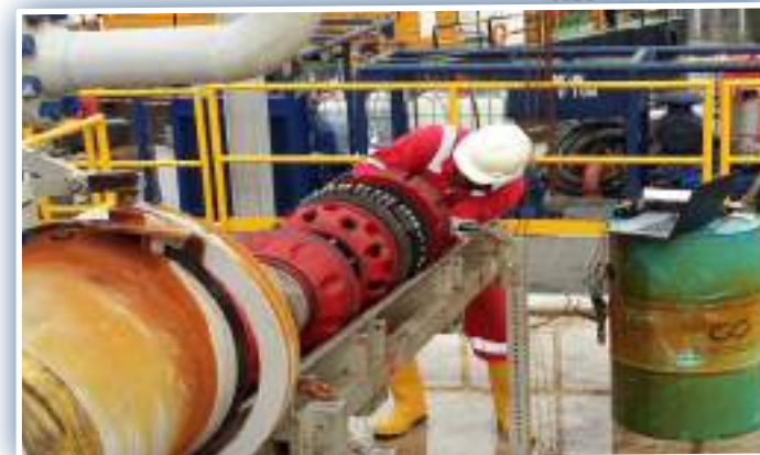
Pipeline Pigging in Progress
