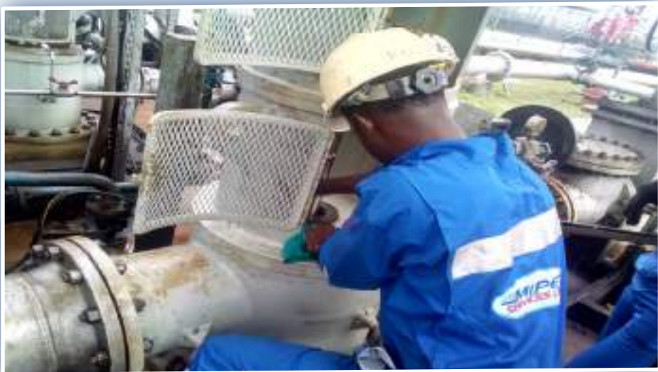
CRUDE OIL TRANSFER PUMP INSTALLATION IN PROGRESS AT UPS (NPDC/SHORELINE FACILITY)
