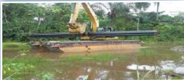
Pipeline Installation across the River
