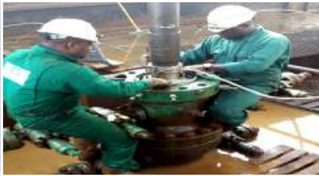
Servicing of WellHead in Progress
