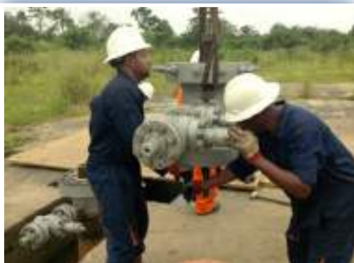
Wellhead Installation in Progress
