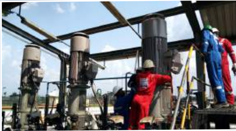
DISMANTLING PROCESS 3 NOS. CRUDE OIL TRANSFER PUMP AT UPS (NPDC/SHORELINE FACILITY)
