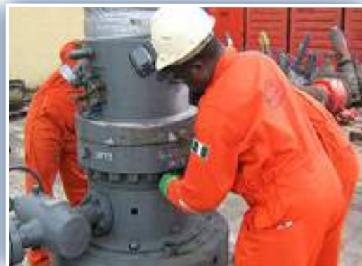
Wellhead Installation in Progress
